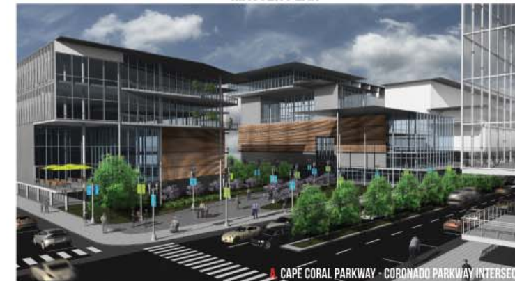
CAPE CORAL PARKWAY - CORONADO PARKWAY INTERSECTION
